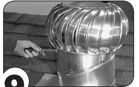
**9** Position the **Whirlybird®** turbine head on the base. Line up the predrilled holes in the brackets and elbow and fasten with sheet metal screws.
