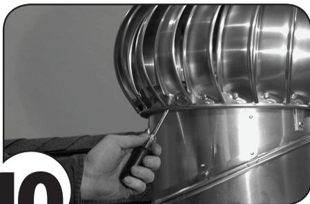
**10** After installing, check to see that **Whirlybird®** turbine vent turns freely. In transportation it may have shifted slightly. If necessary, minor adjustment may be made by gently prying lowest point of turbine upward to remove any wobble.
