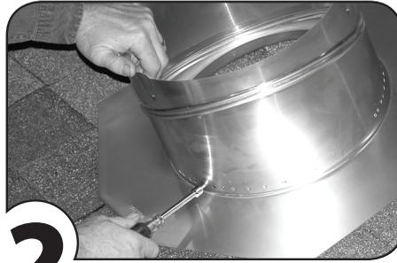
**2** Align roof pitch number on elbow with the indicator line on the base flashing. Place 3 screws through holes that line up with predrilled holes in base.
