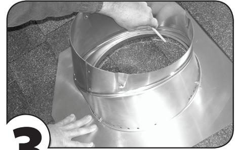
**3** Locate base opening between rafters and mark hole to be cut. Locate rafters by tapping roof.
